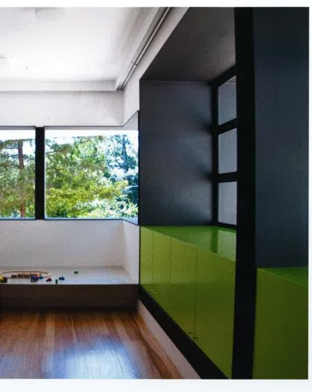
Left: The three modules are integral windows/storage units, constructed from a 10mm steel plate and steel window frames, Below: The new kitchen was placed in almost the same position it had occupied previously.
